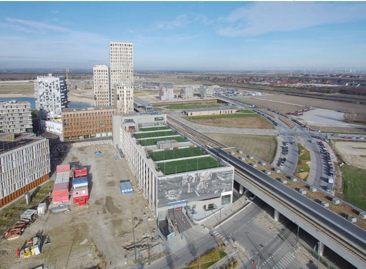
SeeHub-Garage am Baufeld J14C
